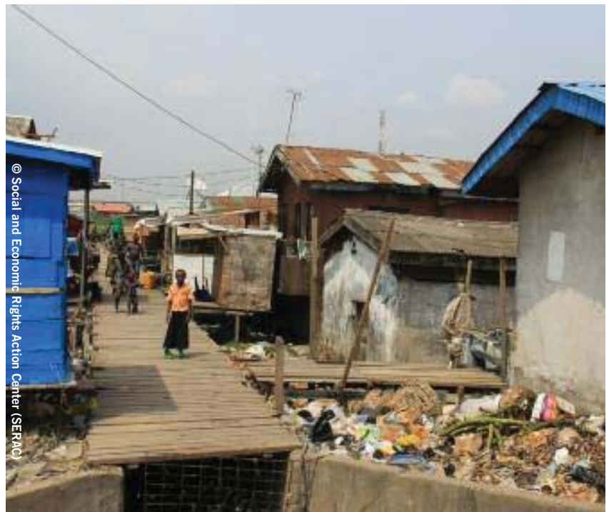
A section of the Badia East community before the forced eviction of 23 February 2013.
