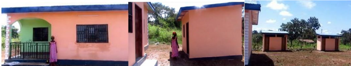
Photo 2: After relocation – from left to right main house, external kitchen, bath + toilet
