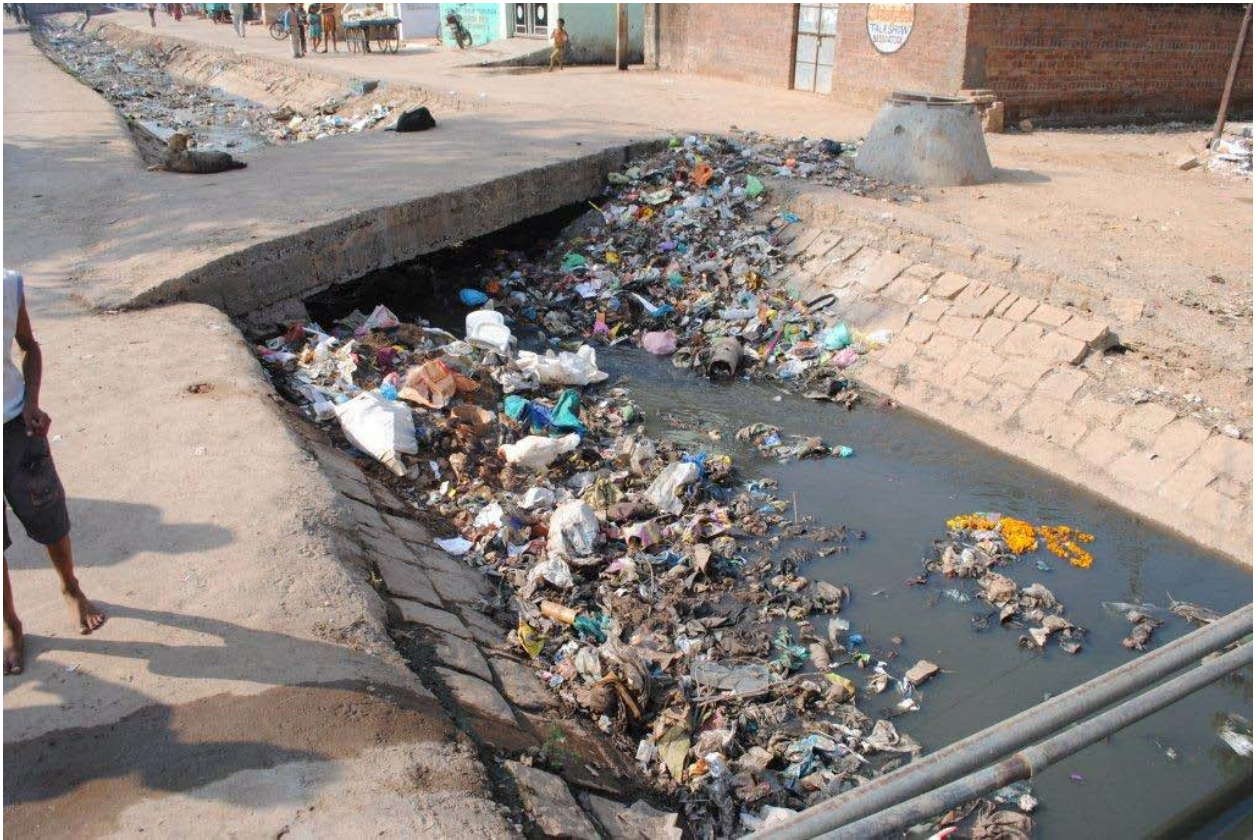
Photo 3. October 2010: Accumulation of debris in a Nalla due to lack of cleaning
