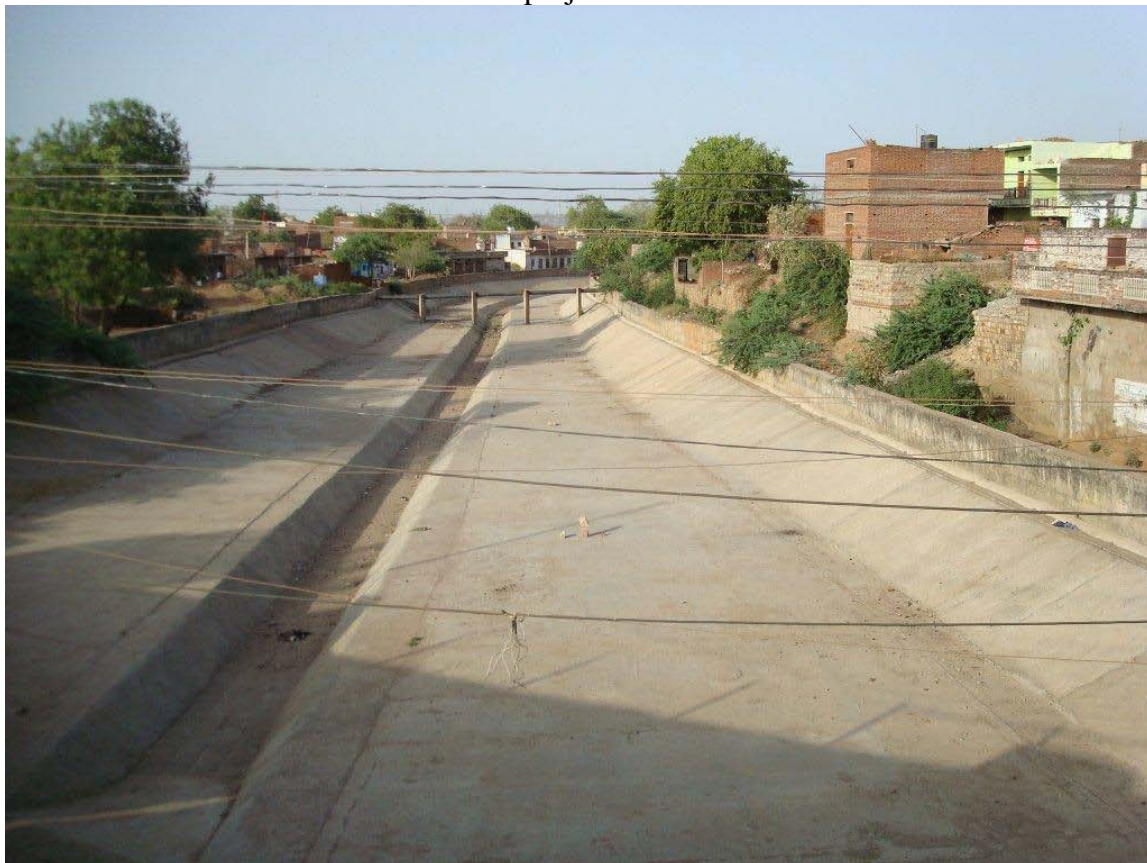
Photo 2. April 2010: Lined river bed after Sub-project intervention
