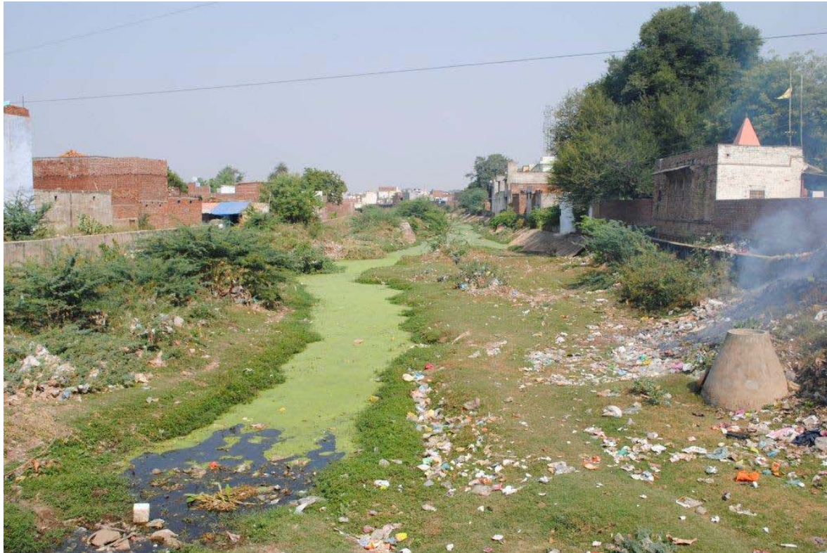
Photo 1. Swarn Rekha River before Sub-project intervention
