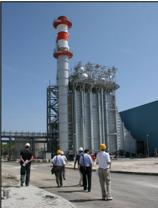
Photo 2. TPP inside facility area
