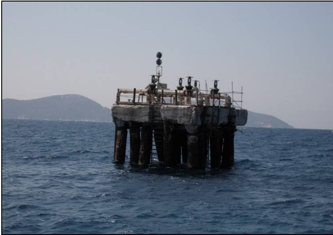
Photo 10. Old oil terminal (not part of project)
