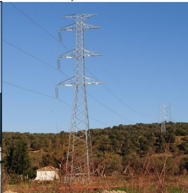
Photo 3. New transmission line
