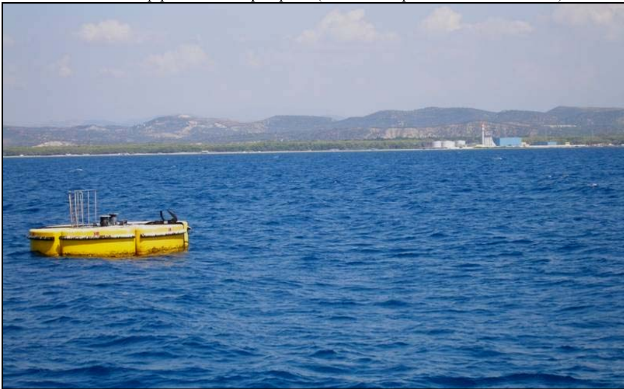
Photo 9. New buoy for securing tanker to off-load fuel; plant in distance
