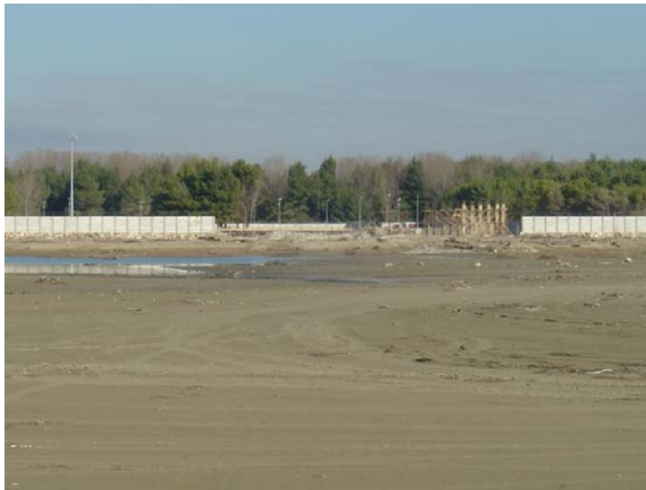
Figure 4 Vlora TPP Construction Site
