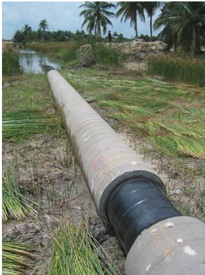
Picture 5: Pipeline with Concrete Coating for Swamp Conditions
