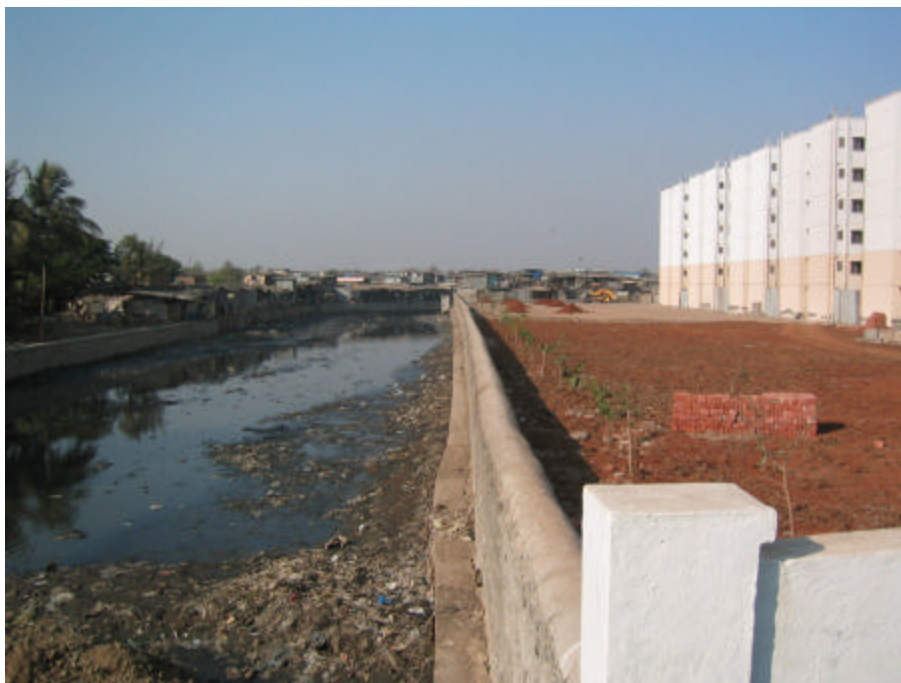
Picture 3.1 Drains along Mankhurd Resettlement Site
