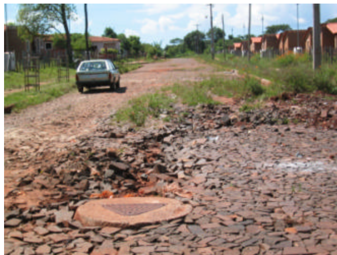
Figure 4 Arroyo Porá Resettlement Site: Poor Quality Construction of Road Recently Built
