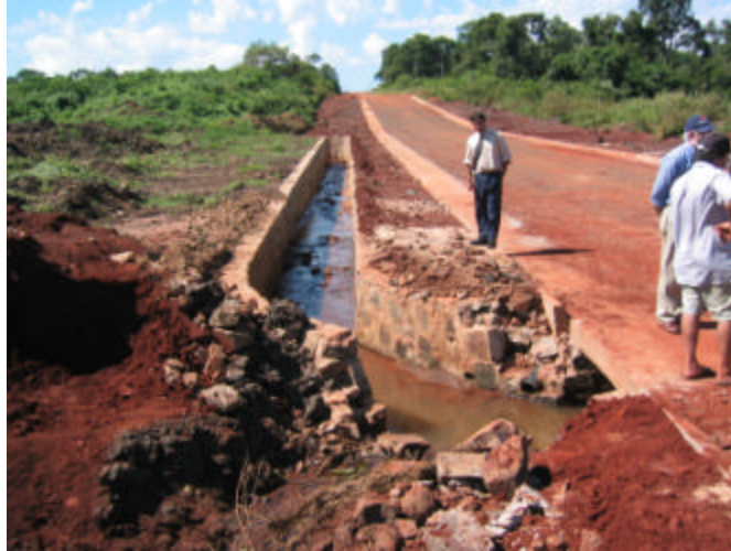
Figure 3 Arroyo Porá Resettlement Site: Inappropriate Design of Drainage Channel
