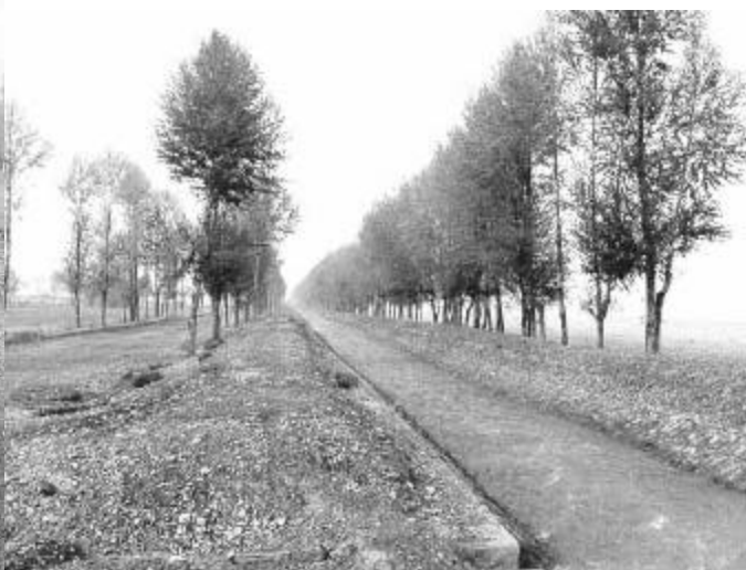
Figure 4b. Canal to prison farm, near Xiangride. Water will be diverted from this canal to irrigate the Proposed Project's Xiaoxiatan Irrigation Sub-district.
