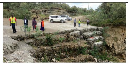
7. KenGen is looking into alternative engineering solutions to address the challenges of flash floods, including the use of check dams
