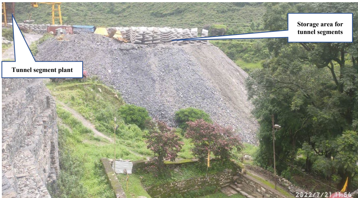
Photo 2. Platform to accommodate the concrete casting plant
