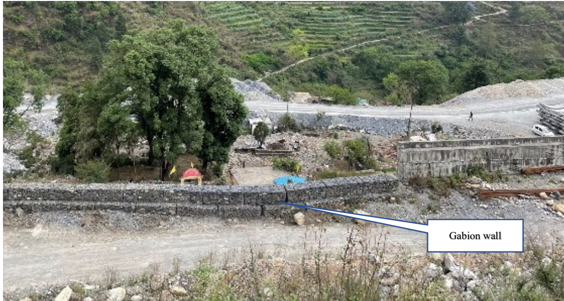
Photo 4. View of the back of the gabion wall (red roof of temple complex visible) showing that no muck is being dumped behind it
