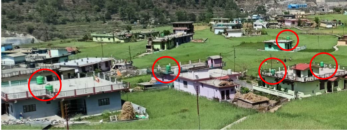
Photo 5: Individual water storage tanks on top of private residences in the Eldana resettlement colony.
