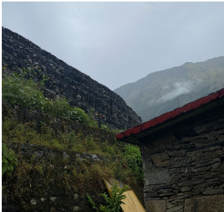
Picture 1: The gabion wall and the Temple's compound wall below it.
