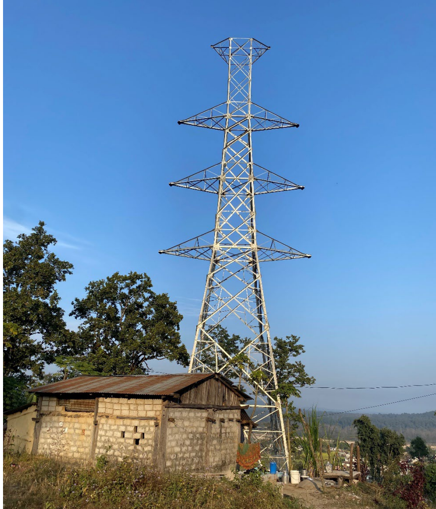
Photo 1. Example of a building (close to tower no. 200) that has to be compensated for and moved
