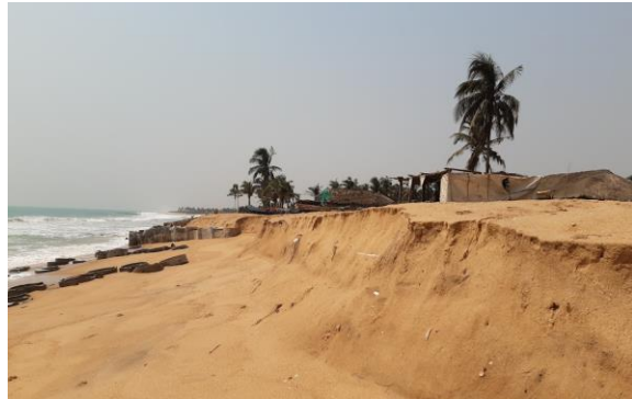
Adissem: view of the Western corridor from its Eastern border
