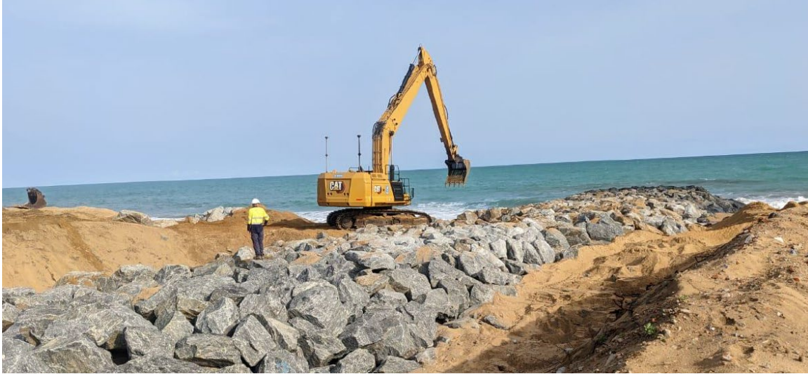
Photo 5. Groyne construction in Togo (March 2023)
