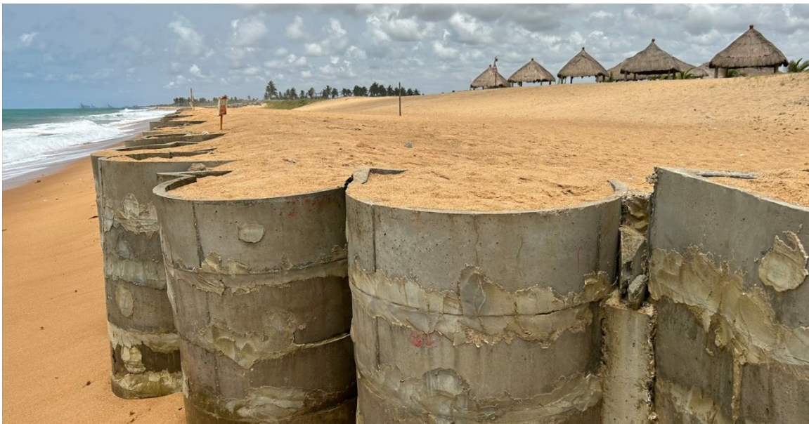
Photo 6. Completed emergency coastal works to protect houses and livelihood assets (March 2023)
