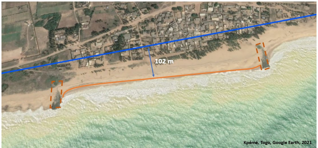
Picture 7. Gain in sand area resulting from groyne construction
