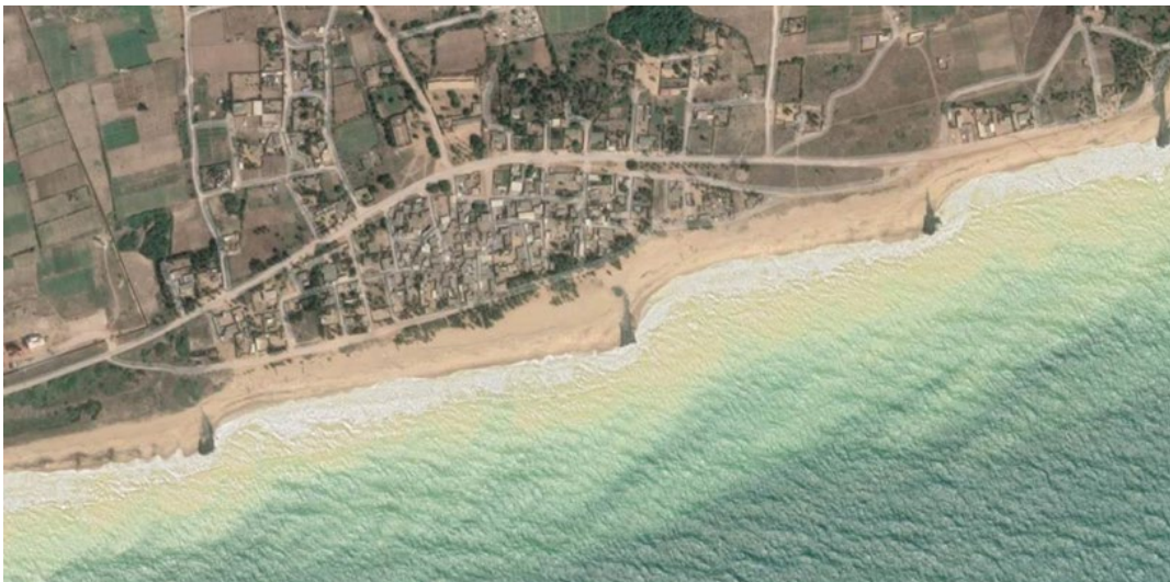
Picture 5. Groynes at Kpeme on the Togolese coast to be rehabilitated by the Project (2021)
