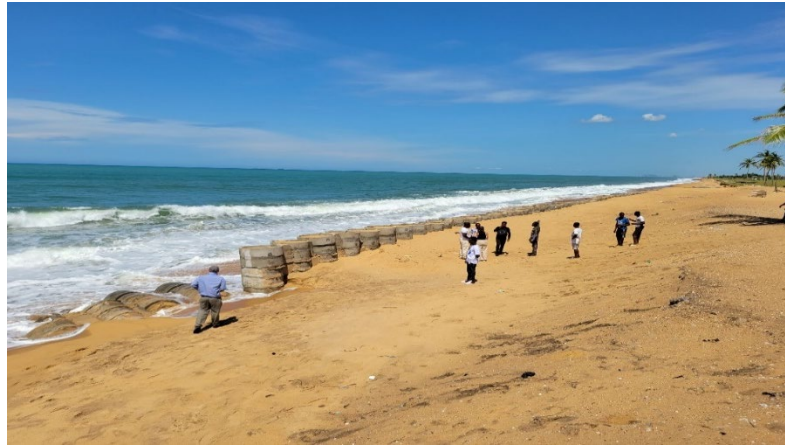
Picture 3: Concrete pipe wall in Tango.
