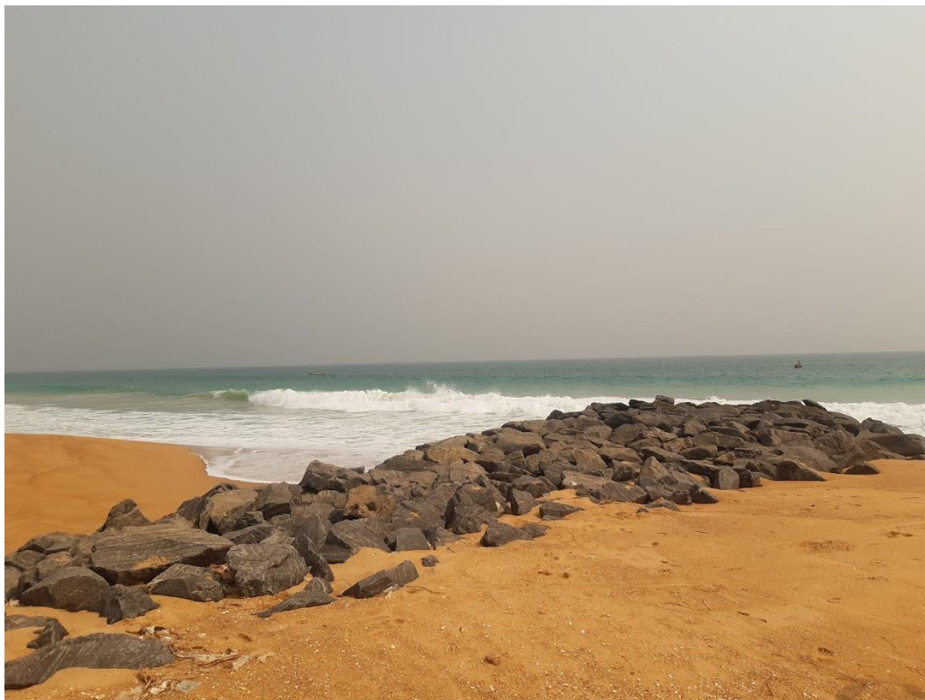
Aného (East Agbodrafo): view of one of the existing protection groynes (construction prior to the WACA intervention)
