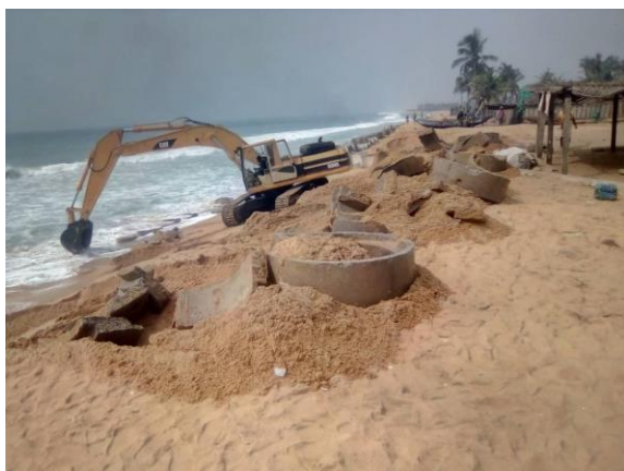
Adissem: excavator in action on 01/28/2022 to remove pipe segments stranded on the foreshore (Contractor photos)
