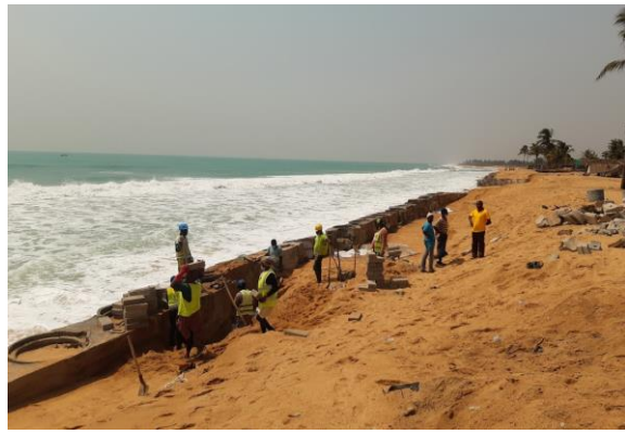
Adissem: central part of the wall being repaired / reinforced
