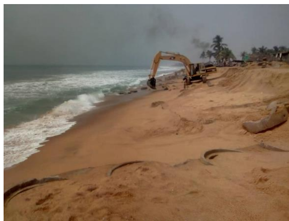
Adissem: excavator in action on 01/28/2022 to remove pipe segments stranded on the foreshore (Contractor photos)
