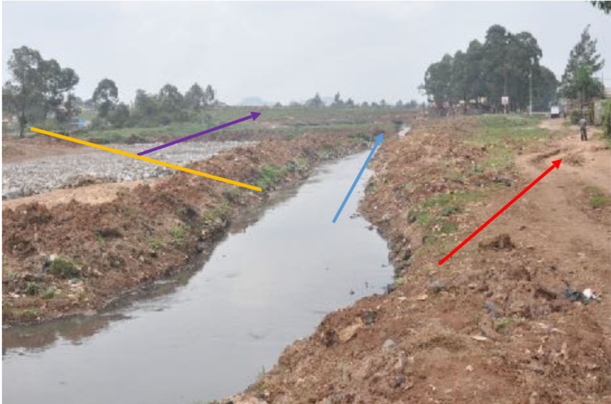
Figure 3 the natural course and the diversion of the channel
