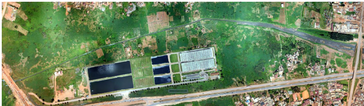
Picture 3: Aerial photo of the Lubigi channel between Kawaala Bridge and Hoima Road (Kawaala-Hoima Section). The Lubigi sewage treatment plant (not part of the Project) is shown south of the channel.
