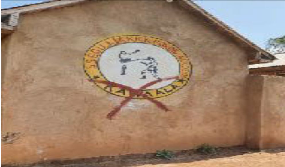
Figure 1 Properties marked for demolition by KCCA officials
