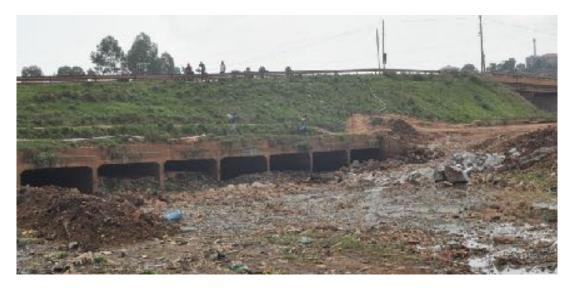
Picture 5: Silting of the box culverts at Kawaala Bridge (2021).
