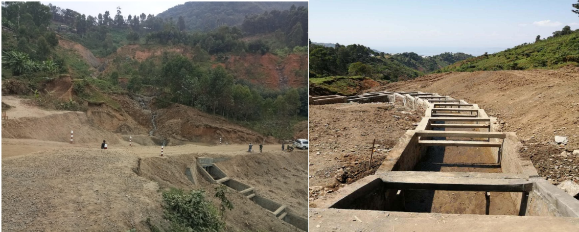
Completed drainage structure at “Chez les Français” on the RN2 Bukavu-Goma road.
